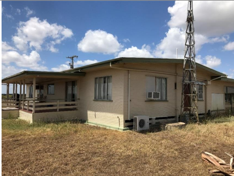
Plate 18-1: ID No. 1: Main farm residence northerly aspect
