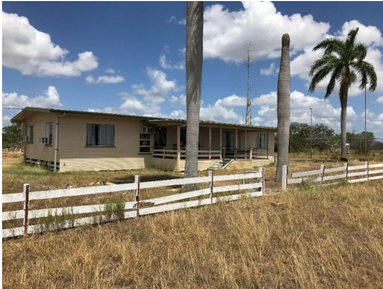
Plate 18-2: ID No. 1: Main farm residence south easterly aspect
