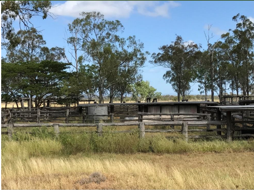
Plate 18-9: ID No. 3: Timber post and slab stockyards
