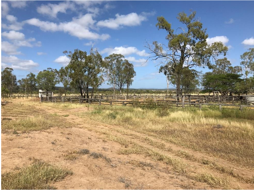
Plate 18-10: ID No. 3: Timber post and slab stockyards
